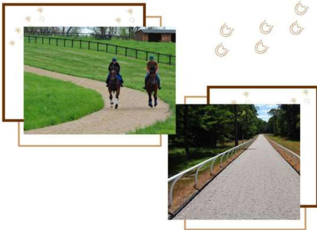
This complete race track system is specifically designed and formulated for horse safety and injury reduction. AmeriTrack is engineered with a free-draining base and all-weather cushion. It incorporates a vertical drainage system which eliminates movement of the cushion to the rail and results in a consistent, no bias track.
